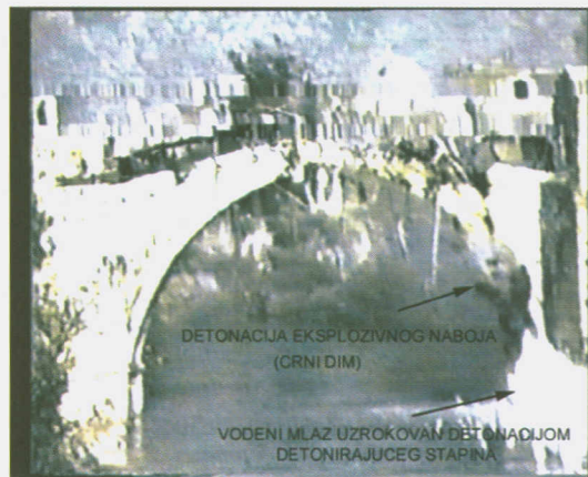
Picture 7 Chronological sequence of the occurrence of the water gush and the explosion at the bottom of the bridge arch.
