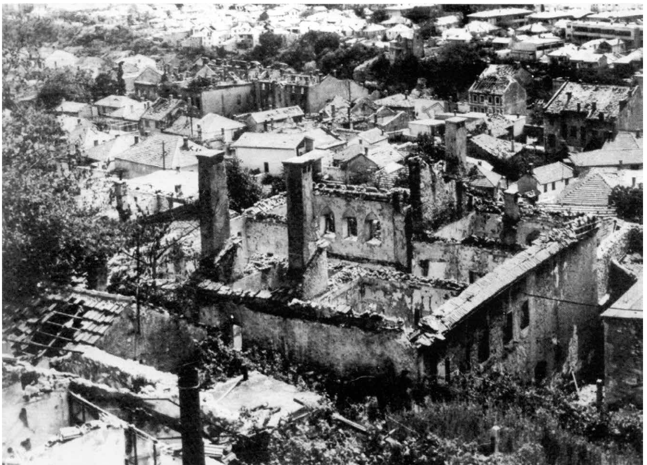
127. View of the left bank of the Neretva, residential district of Luka
