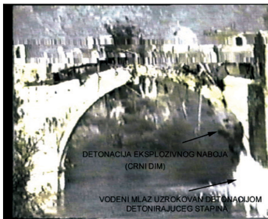
Picture 7 Chronological sequence of the occurrence of the water gush and the explosion at the bottom of the bridge arch.
